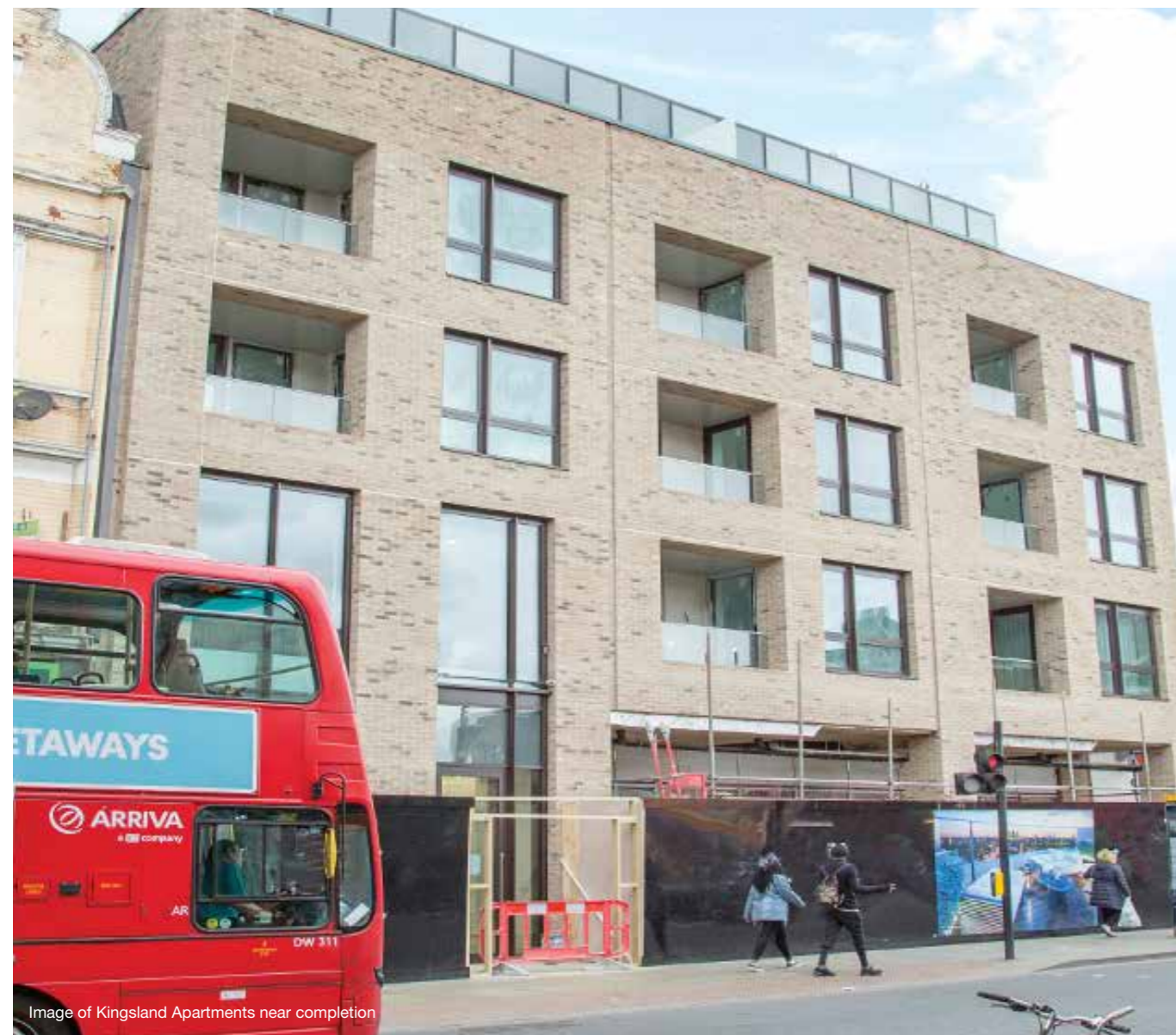
Image of Kingsland Apartments near completion
